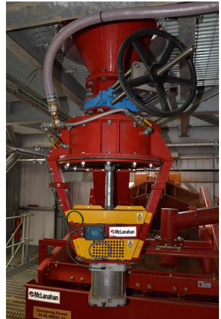
Linear CV “dart” style underflow valve provides hydraulic stability and perfect valve capacity.
